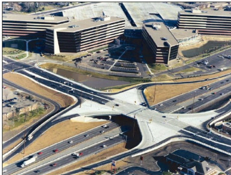
Figure 8 Transportation interchanges can form the basis for public-private partnerships (Source of graphic: ACHD State Street Corridor Study)
